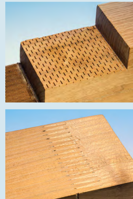
Above: Surface structuring by means of lasers improves the bonding of glued laminated timber made of Robinia.
